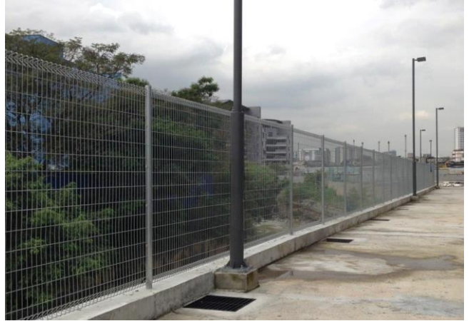
Anti Climb Perimeter Fencing
